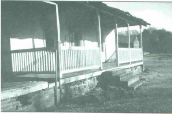
New porch on original front of home with cypress planks & hand trimmed nails.
